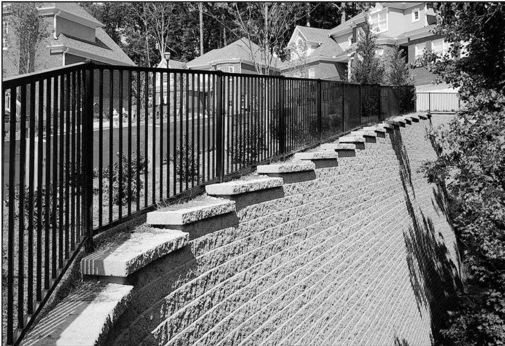
Often fences, stair rails, guide rails, or concrete traffic barriers are needed behind a VERSA-LOK wall. With proper design and installation, a variety of structural and aesthetic features can be placed at the top of a VERSA-LOK wall.
